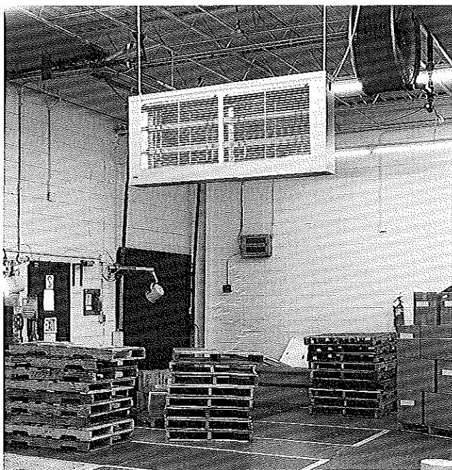
Figure 1. A blacklight trap with electrocuting grid, suitable for all flying stored-product moths and beetles.
